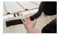
Start from the end of the ridge, rolling out VistaVent universal venting material along the length of the ridge (both sides), making sure the bottom edge of the venting is 1/2"-1" up-slope from the edge of the ridge cap.
