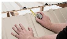
Make sure panel is free of dust and debris. If not pre-cut, cut 2" slot at ridge. Measure and mark where the ridge cap will sit on the panel.
