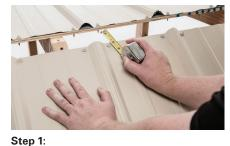
Make sure panel is free of dust and debris. If not pre-cut, cut 2" slot at ridge. Measure and mark where the ridge cap will sit on the panel.
