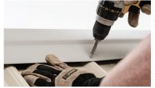
Apply ridge cap, compressing material between the ridge cap and major rib. Fasten at the major rib using an appropriate screw
